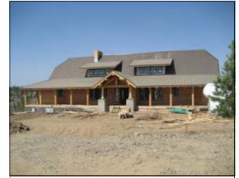
Hawk Creek Estates Club-house under construction
